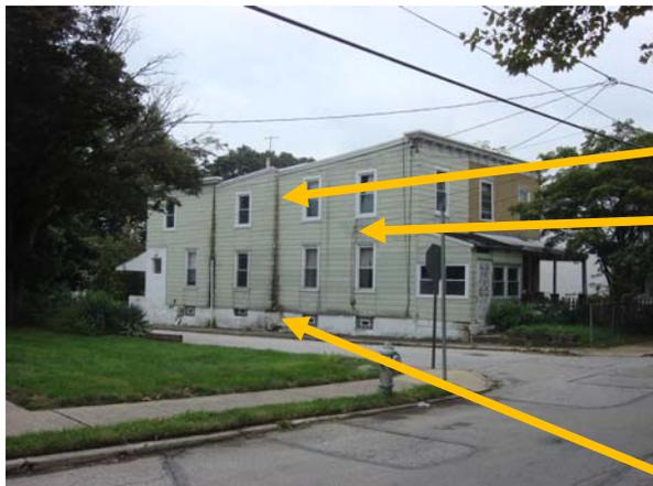
Water draining on side of building, water around windows and water degrading the foundation
