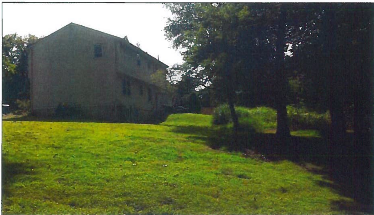
Side / Rear Elevation – Looking South
